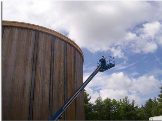
Potter Hill Tank Construction, 2007
